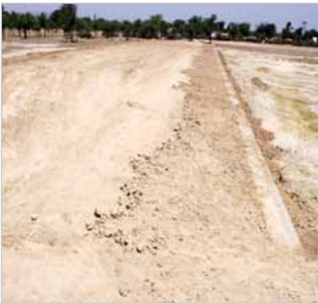
Completed pond- Dansrolii
