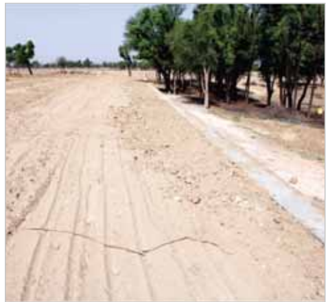
Completed Pond –Kankra
